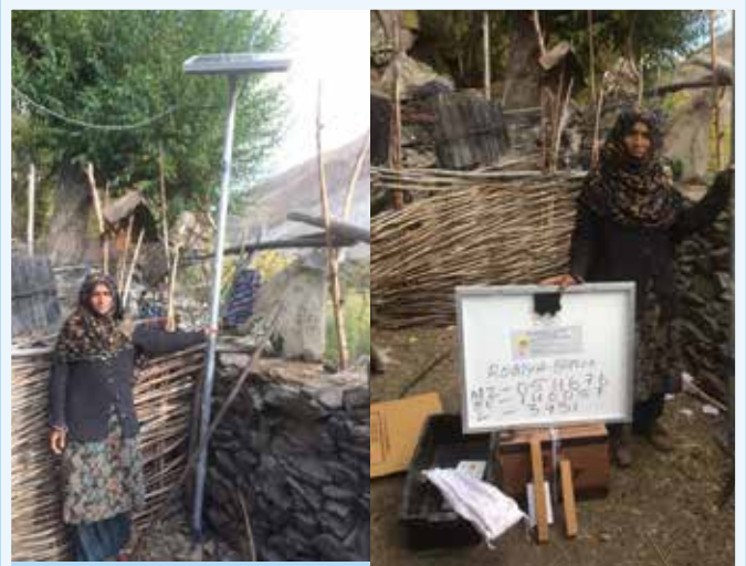
Installation of Solar Photo Voltaic systems in villages of Leh & Kargil
