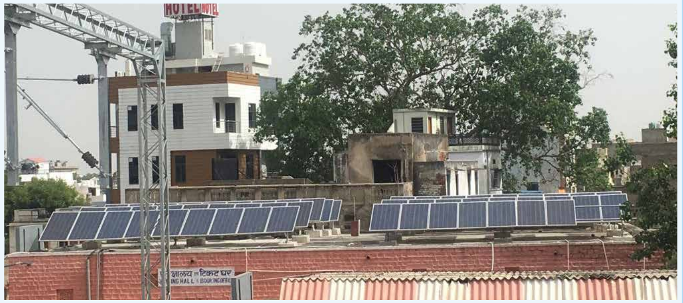
Installation of Solar Panels at Phulera Railway Station
