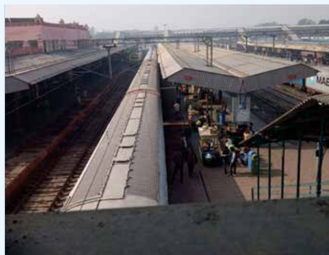
Installation of Roof-Top Solar Panels on Non-AC Railway coaches.
